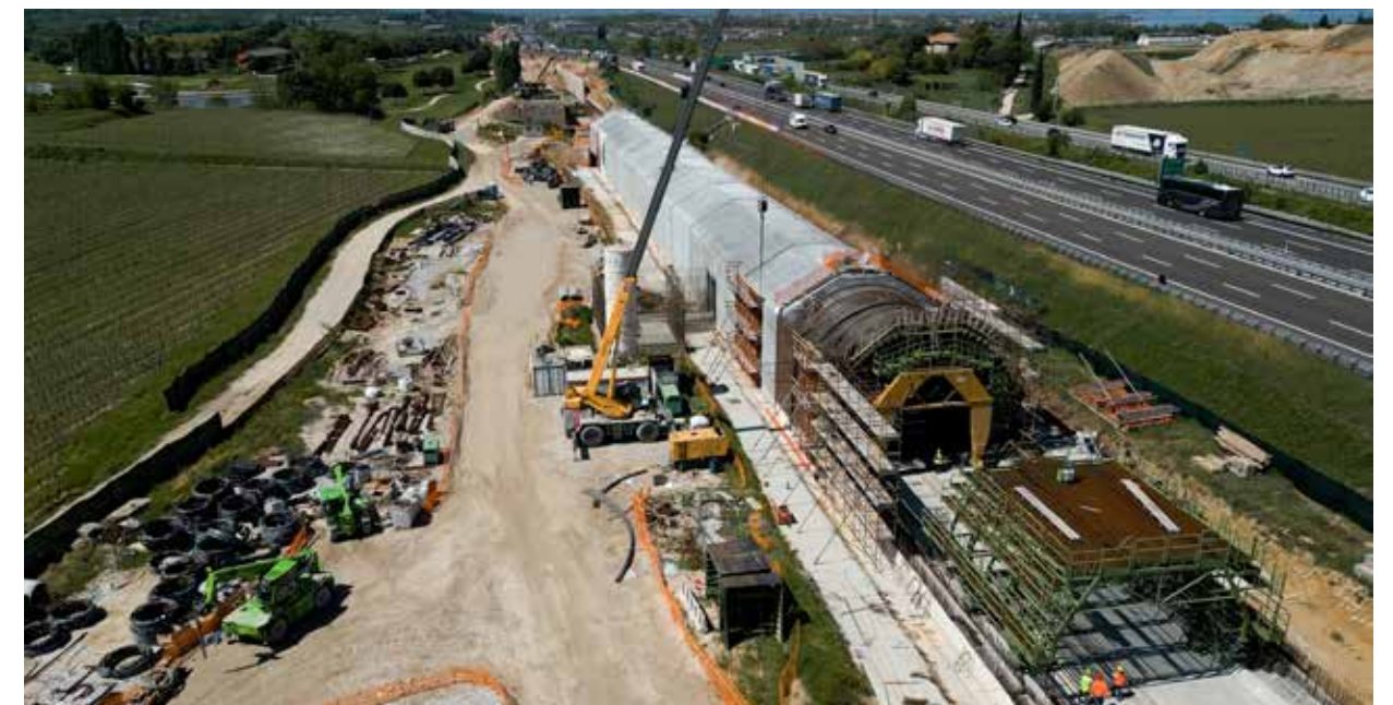
Ferroberica's construction yard - The artificial tunnel for the Bresca-Verona High-Speed train line in Peschiera del Garda (VR)
