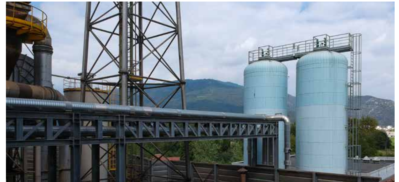
Alfa Acciai: array of pipes supplying the heat recovery plant from the steel mill and storage tanks
